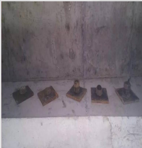
附墙固定垫块尺寸小于100mm*100mm*10mm，且 螺栓外露丝扣小于3丝
