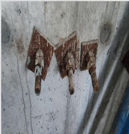
附墙固定垫块尺寸小于100mm*100mm*10mm，且 螺栓外露丝扣小于3丝
